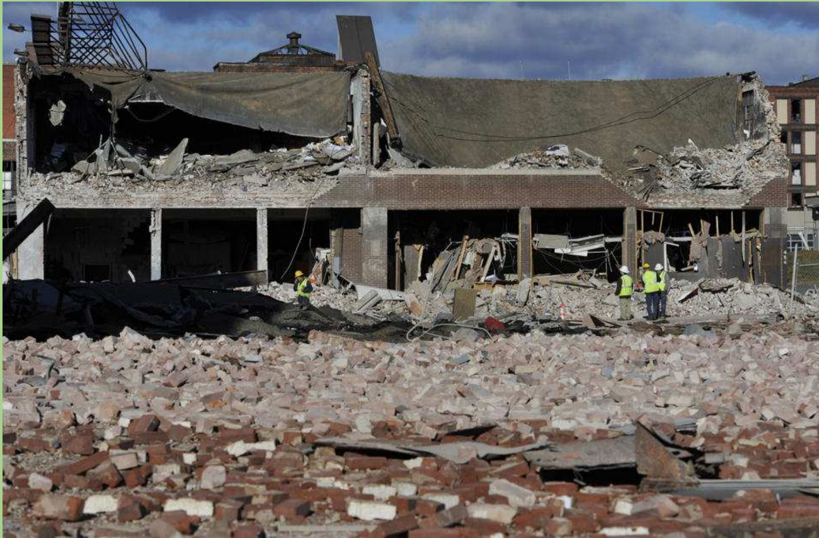
Gas explosion - Springfield, MA - November 23, 2012 over 60 downtown buildings damaged or destroyed
